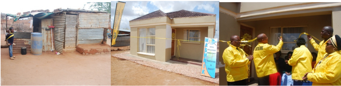
1 st & 2 nd pictures: The Mehale house before it became a home. 3 rd picture: MEC Soviet Lekganyane and Mme Mothibi- Mayor of Mokgalakwena Municipality looking on as Chief Matlala cuts the ribbon to declare the official hand-over to the family
